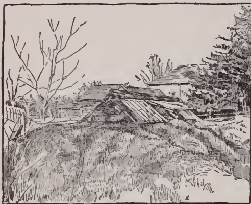
2742. The roof of No. 4. Fig. 2741.
